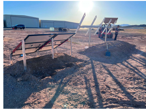
PHOTO 2: Horizontal force test setup
