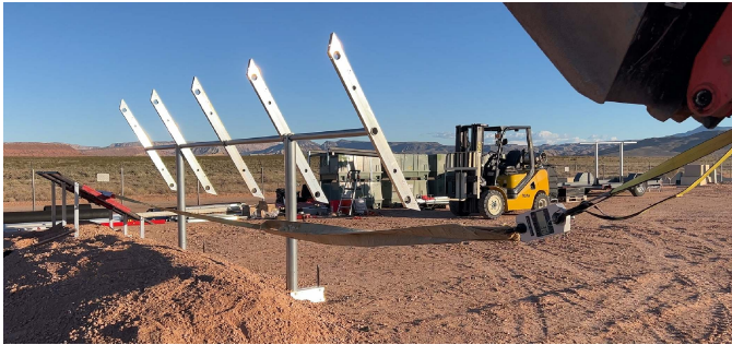
PHOTO 1: Horizontal force test setup
