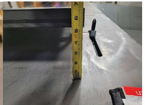
Figure 6: Height from roof to panel, Runs 2 & 3
