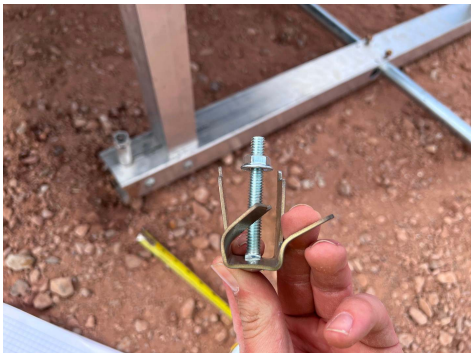
PHOTO 13: Bracket deformation after testing
