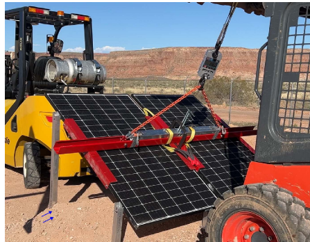
PHOTO 5: Test 1 - Evidence of ballast shift
