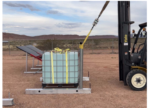
PHOTO 3: Load applied at ~ 60 degree angle.
