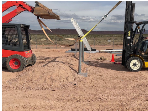
PHOTO 2: Frame under load
