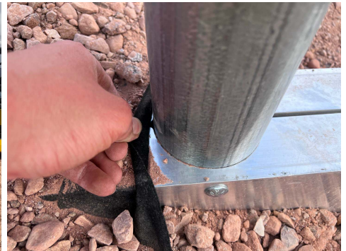
PHOTO 3: No signs of deformation observed after testing
