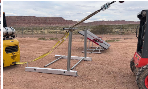
PHOTO 5: 3 rd test under load
