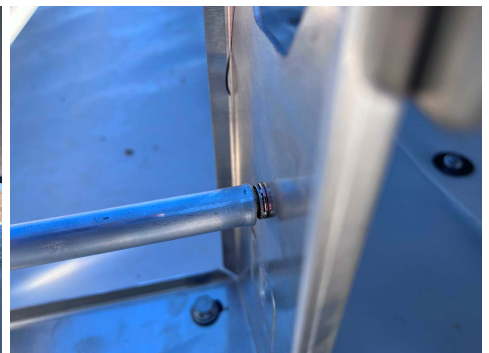
PHOTO 9: Rivnut slip / failure
