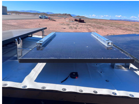
PHOTO 2: Setup with no load and aluminum distribution bars in place
