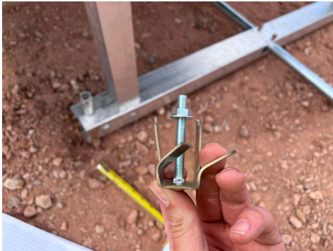
PHOTO 13: Bracket deformation after testing
