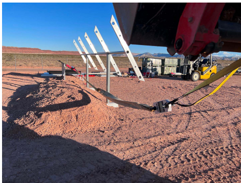
PHOTO 3: Horizontal force test setup
