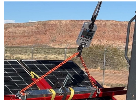
PHOTO 6: Test 1 - Load at ballast shift
