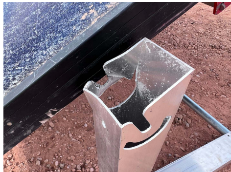
PHOTO 14: Upright mount deformation after testing
