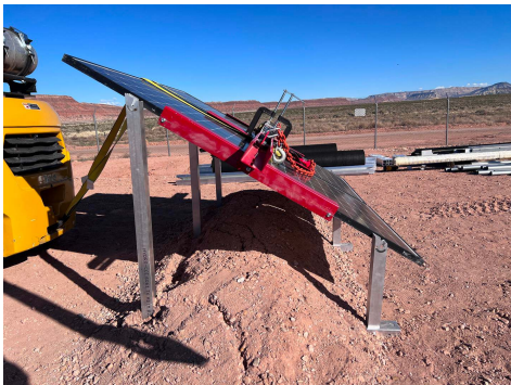
PHOTO 13: Ballast after completion of testing
