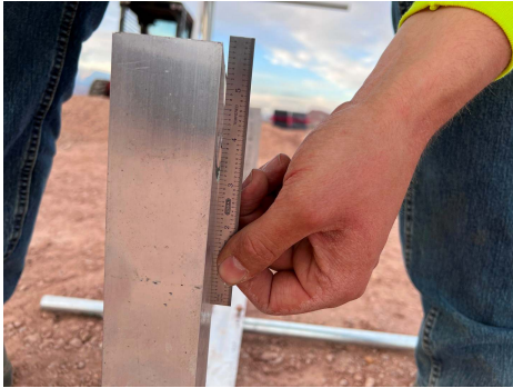
PHOTO 10: Slight deformation after load removed
