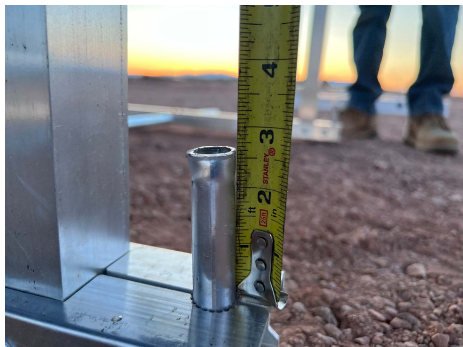
PHOTO 4: 'Stickout' measurement example at Spike #3
