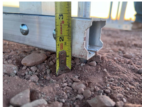
PHOTO 5: Ground to frame measurement example at Spike #3
