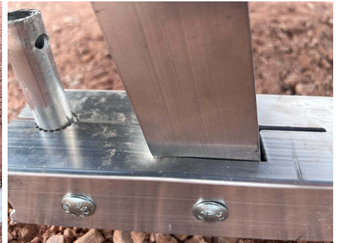
PHOTO 15: Upright deformation after testing
