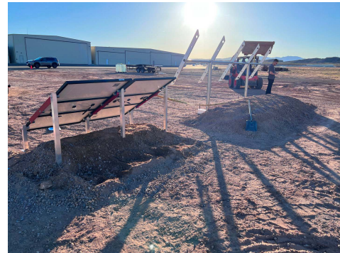
PHOTO 2: Horizontal force test setup
