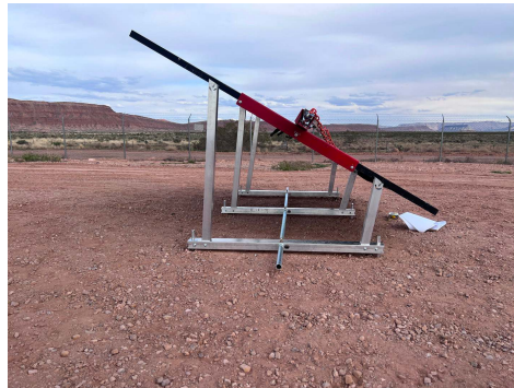
PHOTO 11: Frame after testing
