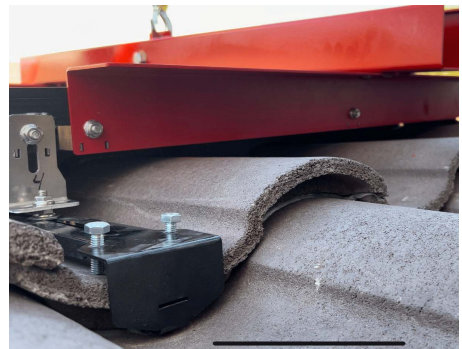
PHOTO 7: Bracket under test load
