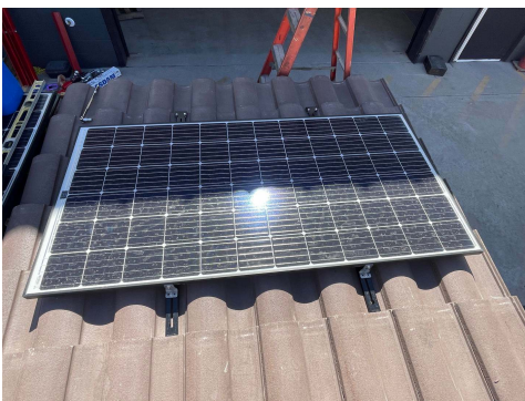
PHOTO 1: Overview of solar panel and tile roof deck - before tests
