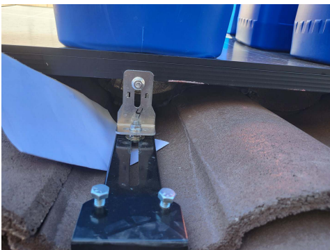
PHOTO 4: Load 1 - Bracket under load
