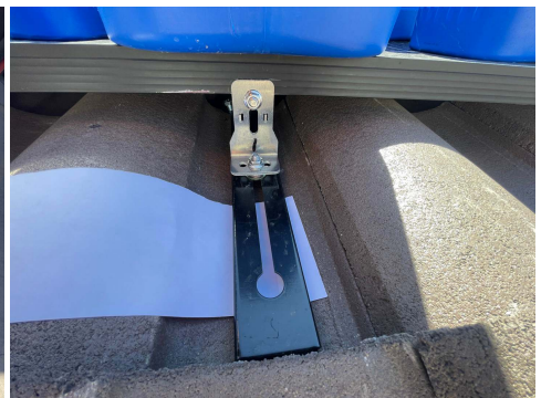
PHOTO 6: Load 2 - Bracket under load
