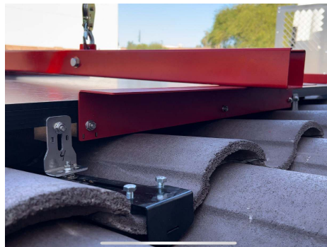
PHOTO 8: Bracket unloaded after test
