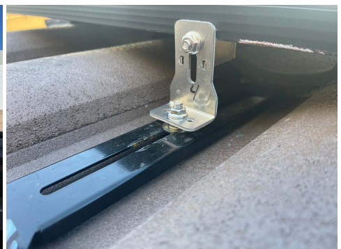
PHOTO 9: Unloaded Bracket - after tests
