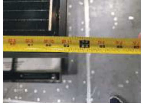
Figure 21: Solar panels total length 83 in.
