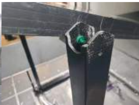
Figure 17: IR Ballast frame connection to solar panel
