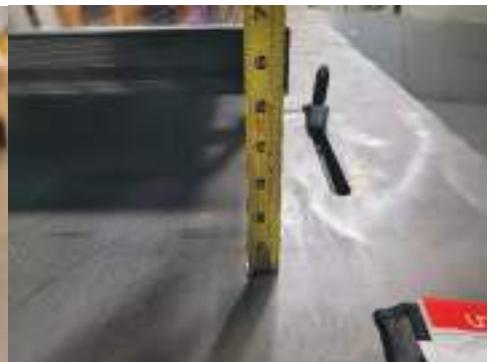
Figure 6: Height from roof to panel, Runs 2 & 3
