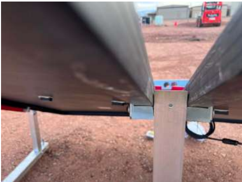
PHOTO 12: Middle brackets after testing
