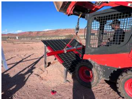
PHOTO 4: Test setup with dynamometer and chains connected
