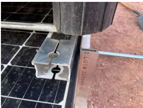
PHOTO 7: Slight deflections noted under load
