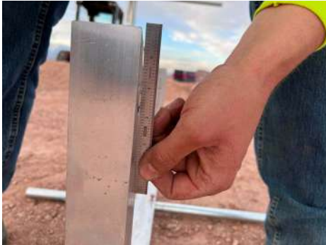
PHOTO 10: Slight deformation after load removed
