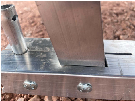
PHOTO 15: Upright deformation after testing
