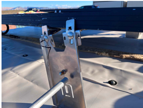
PHOTO 5: After cross-member disengagement
