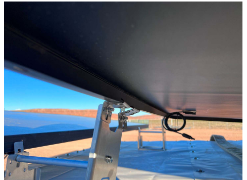
PHOTO 6: After cross-member disengagement
