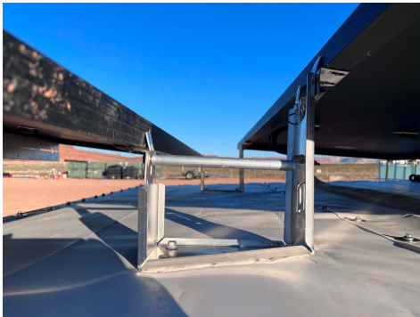
PHOTO 4: After cross-member disengagement
