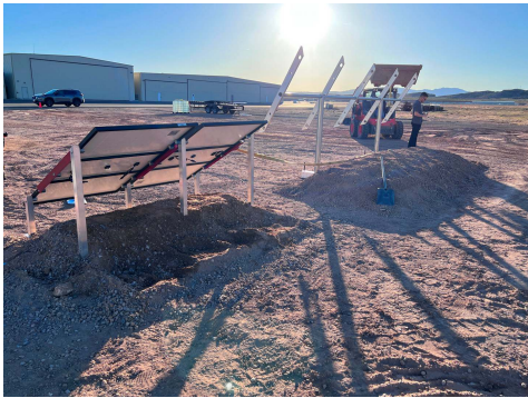
PHOTO 2: Horizontal force test setup
