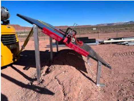
PHOTO 13: Ballast after completion of testing
