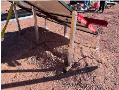
PHOTO 14: Ballast and frame after completion of testing
