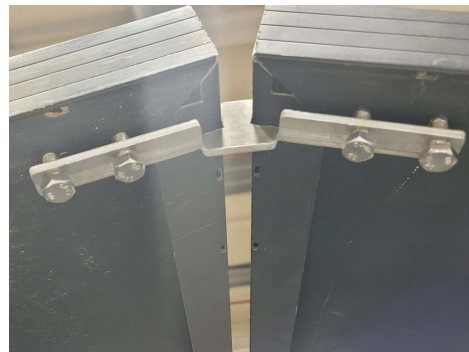
Photo 12: Underside of panel at ridge prior to testing.
