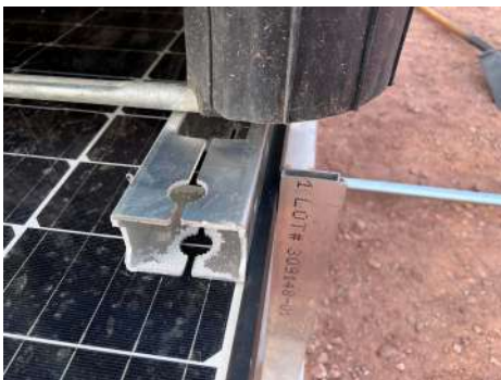
PHOTO 7: Slight deflections noted under load
