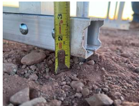
PHOTO 5: Ground to frame measurement example at Spike #3
