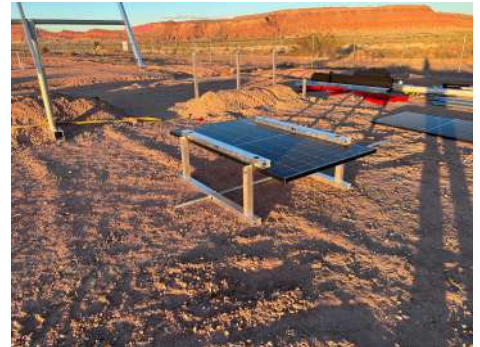
PHOTO 3: IR-30 Solar Racking System setup for test
