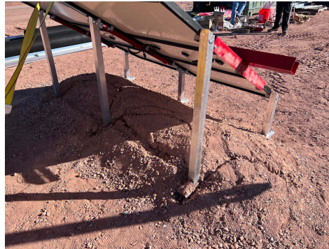
PHOTO 14: Ballast and frame after completion of testing
