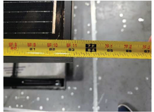
Figure 21: Solar panels total length 83 in.
