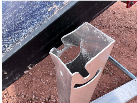
PHOTO 14: Upright mount deformation after testing
