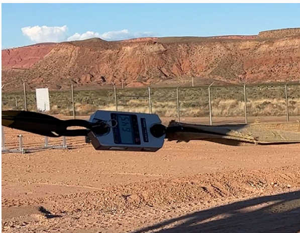
Photo 4: Horizontal force test max load
