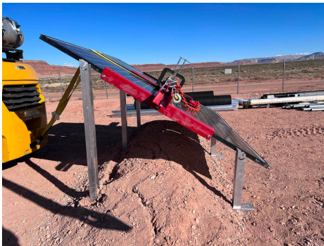
PHOTO 13: Ballast after completion of testing
