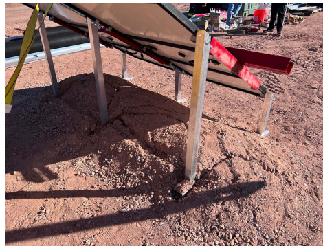
PHOTO 14: Ballast and frame after completion of testing
