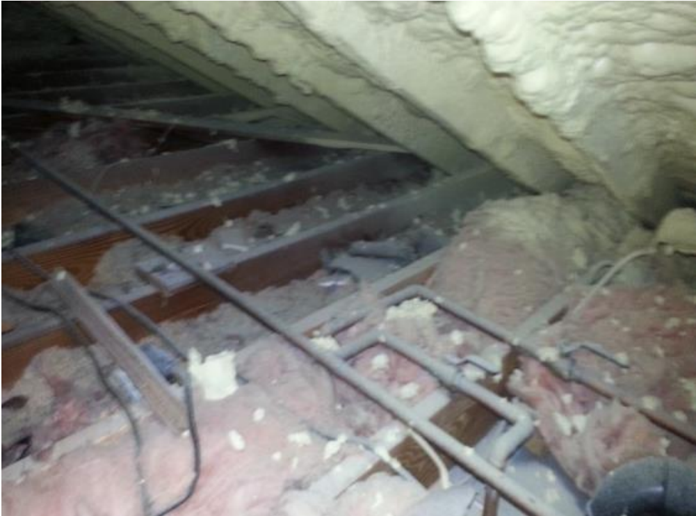
Insulation remaining on floor
