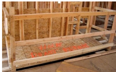
Covered floor hole marked, and with a guardrail surrounding it.
