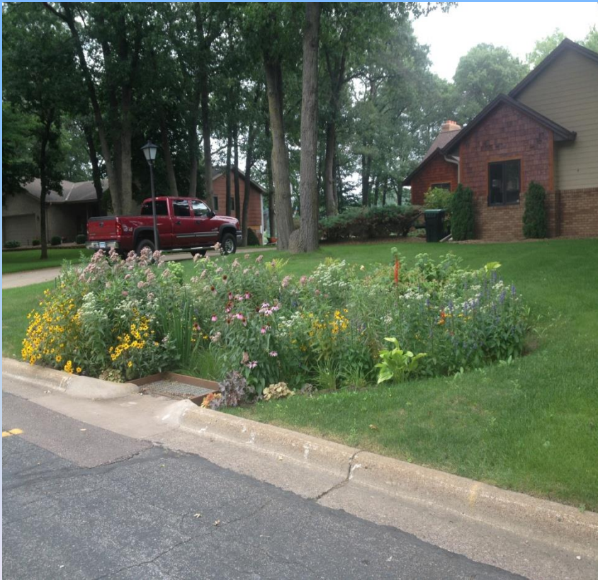
Resident 2: curb cut garden with Rain Guardian installed. 5yrs later
