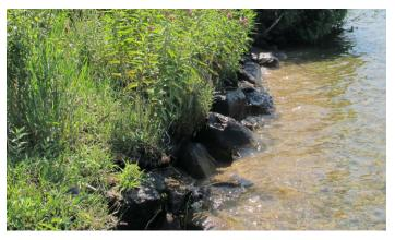
This encapsulated soil lift and the established native shoreline vegetation stabilize the shoreline – even with moderate to high wave and ice action. Encapsulated soil lifts also slow runoff from upland areas, improve fish and wildlife habitat, improve water quality, and deter geese from damaging property. Photo courtesy of Michigan Natural Shoreline Partnership.
