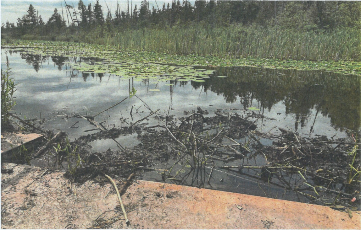
Some debris upstream of the fixed crest wier, not obstructing flow
