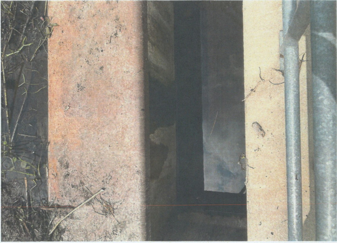
Some seepage observed on downstream side of SSP cap, minor
