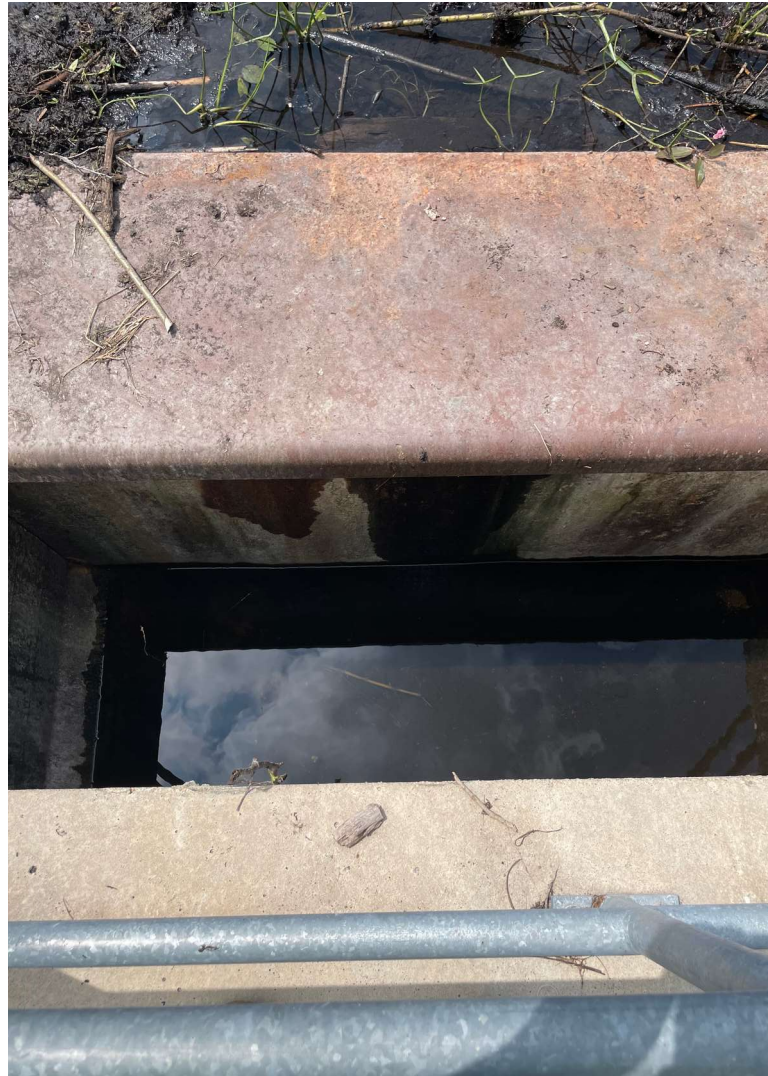
Some seepage observed on downstream side of SSP cap, minor
