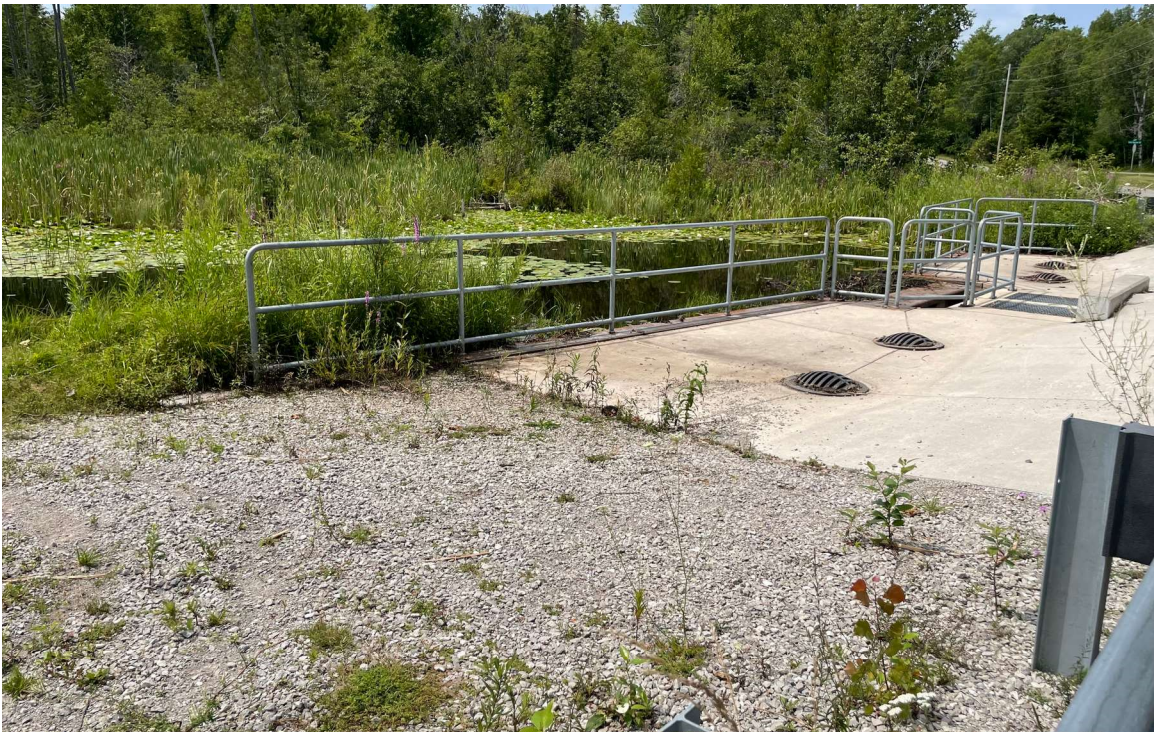
Gravel parking area on right side of dam, new handrail on upstream side of structure
