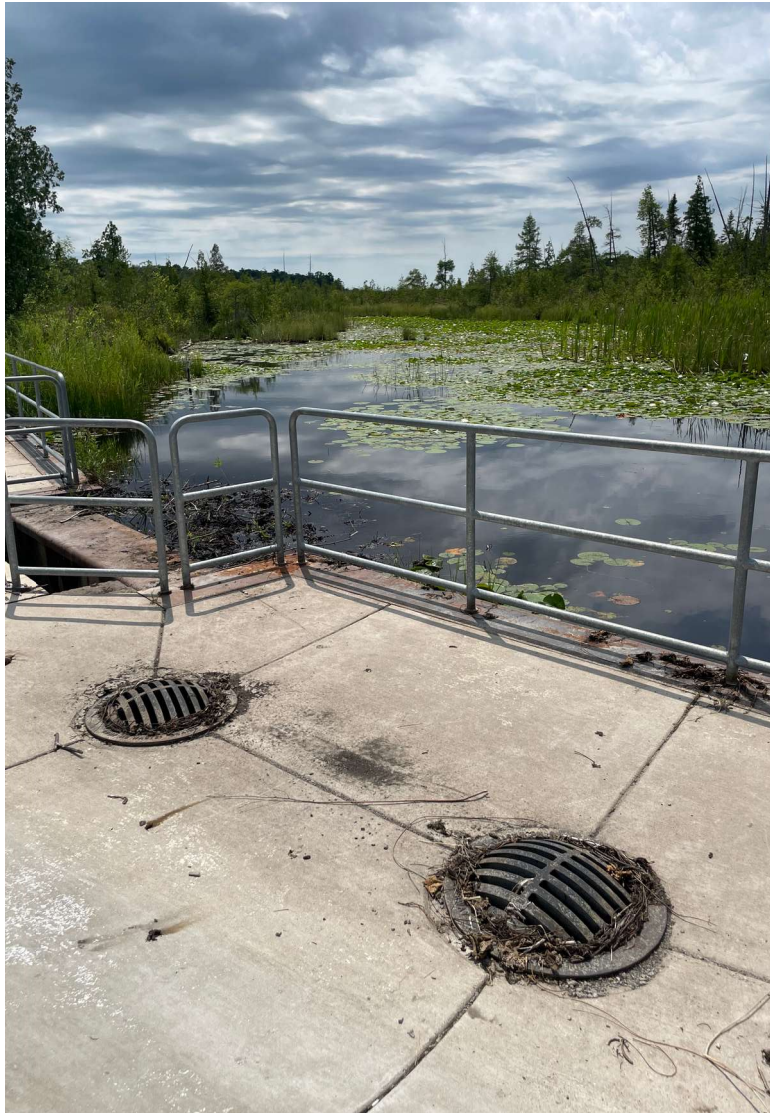
Overflow catchbasin on left side of structure
