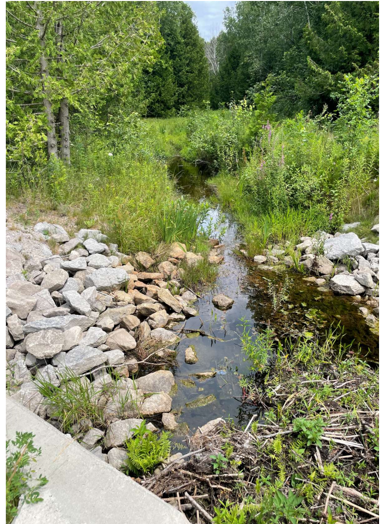
Downstream channel - some brush and mud in flow channel
