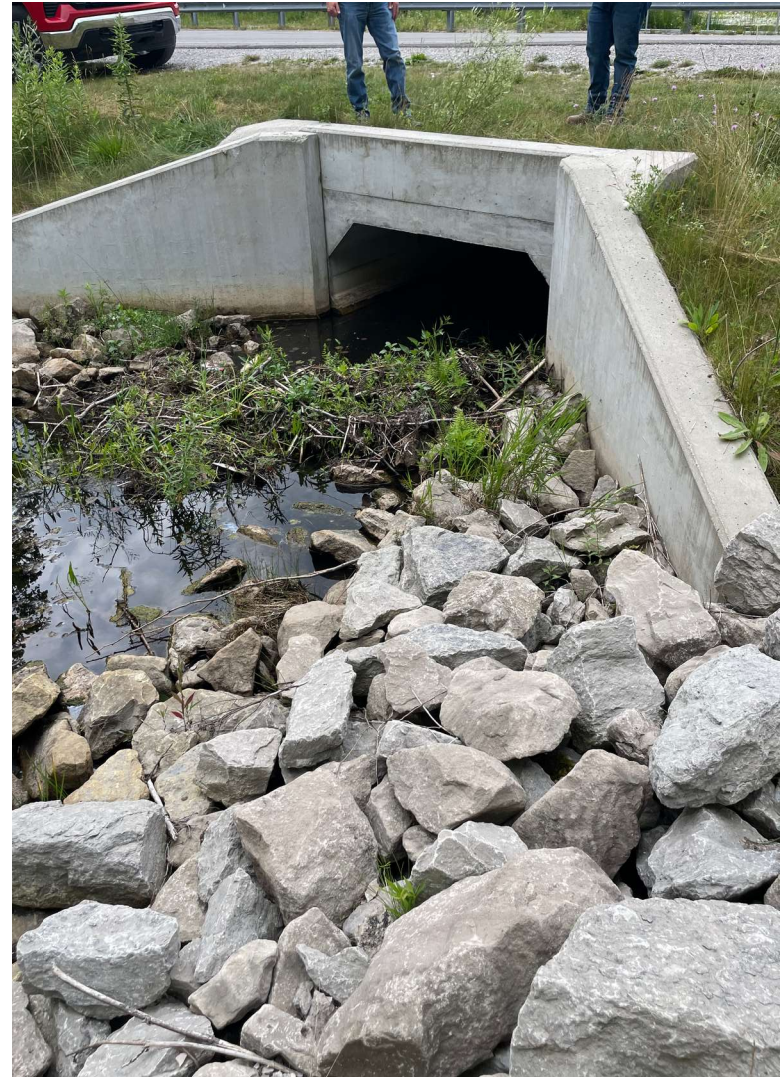
Downstream wing wall, some vegetation on right side wing wall
