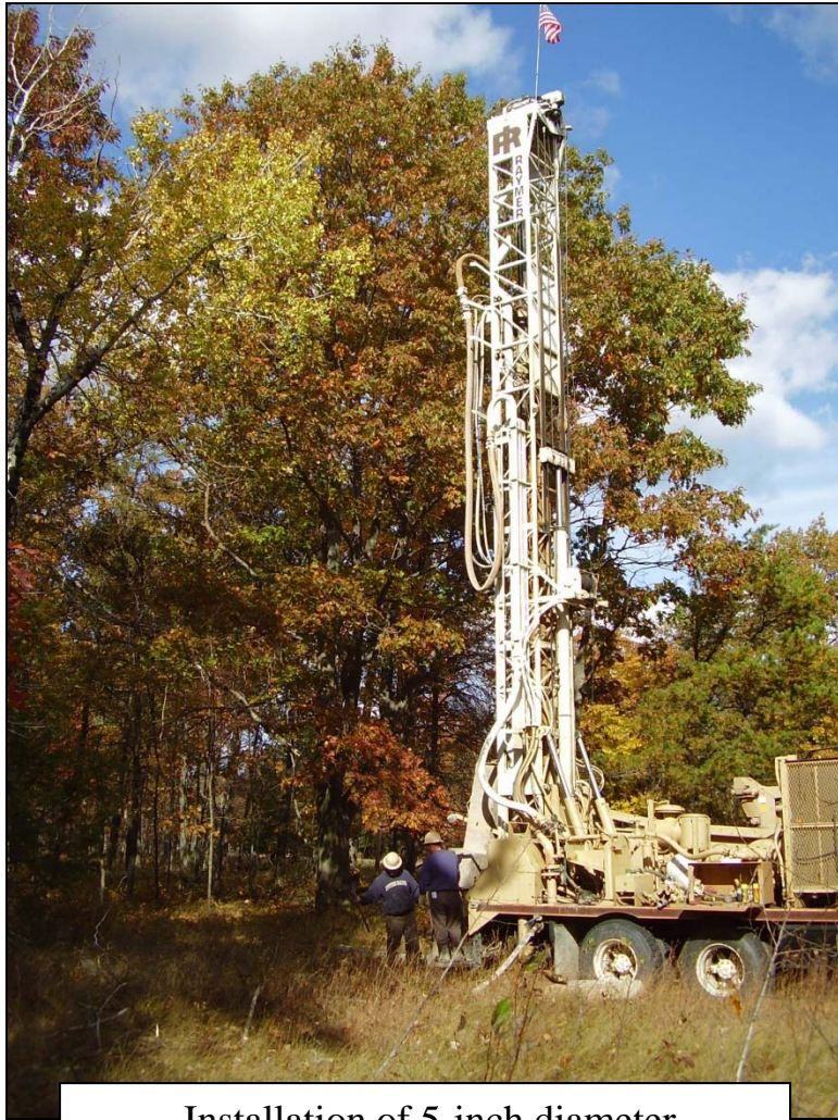
Installation of 5-inch diameter observation well, October 18, 2010.
