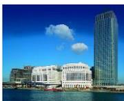
**Canary Wharf Buildings**, Phases II & III, London, England. Provided structural design of five new buildings, two of reinforced concrete and three steel-framed structures, each 12 stories high with two levels of underground parking supported on pile foundations. Also completed preliminary design for two steel-framed highrise buildings (48 stories and 22 stories).
