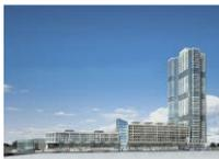
**Columbus Towers Complex, Jersey City, New Jersey.** This project includes the design of a 35-story concrete residential tower (42,000 m<sup>2</sup>), a 7-story concrete parking structure (33,000 m<sup>2</sup>) with a rooftop recreational area including a pool, and a 3-story steel office building (3,400 m<sup>2</sup>).
