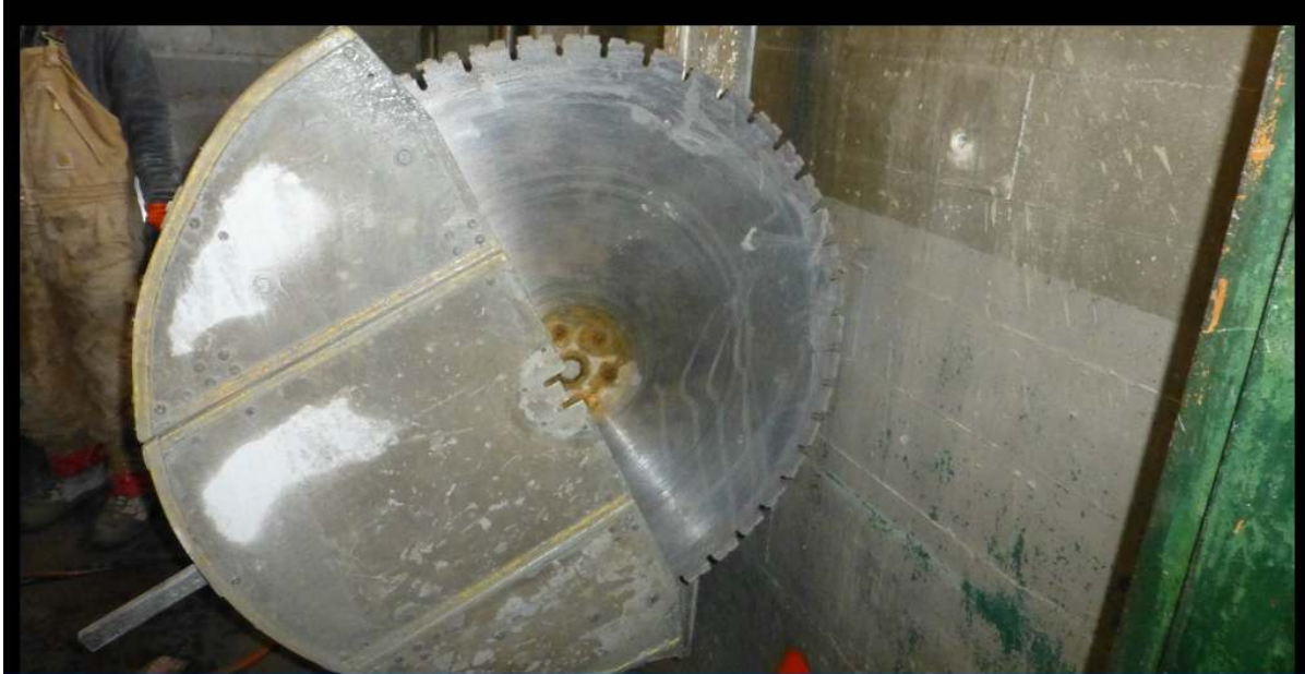
Cut concrete wall for widening window
