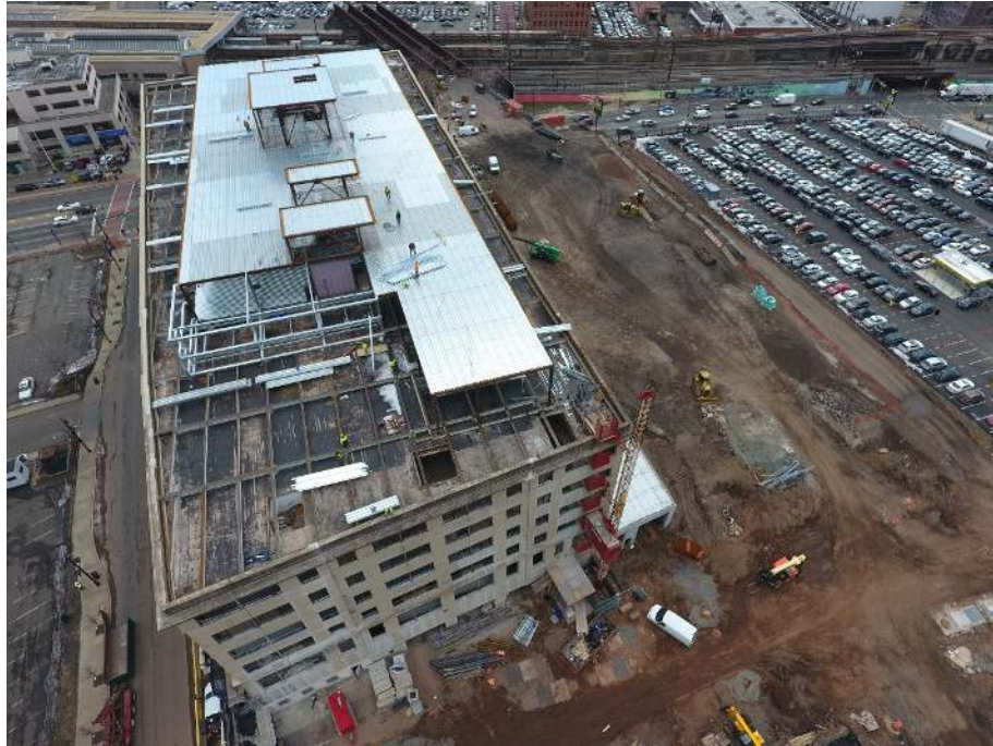
3D Drone View for. New roof framing and penthouse roof
