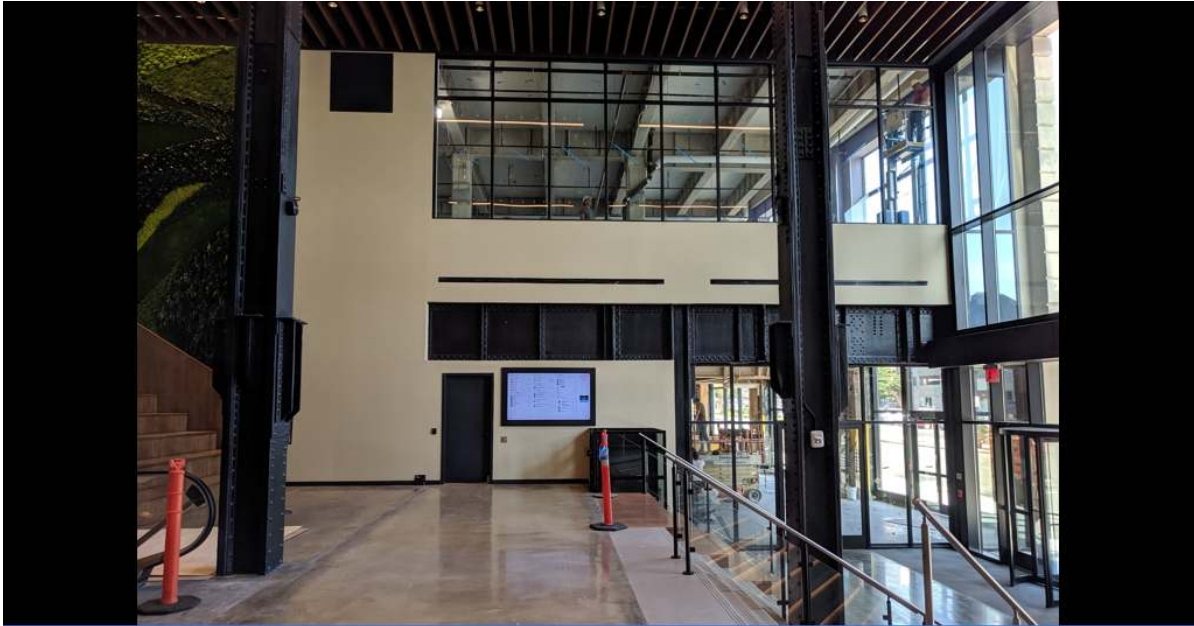
New Main entrance lobby
