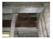
**Structural Investigation at the Rear of the Building,** 163 West 48<sup>th</sup>. Street, New York, New York. A long-time Client that maintains an existing commercial building on West 48<sup>th</sup> Street experienced deterioration of the rear wall of the structure. The vertical face of the wall has bulged and has been short by a number of years. ADG provided Structural Engineering services to evaluate the construction of the building and to prepare a report of our findings.
