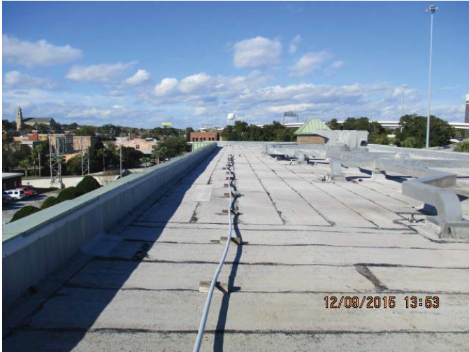
#2 - Predominate Roof Covering - Doesn't Meet 2001 FBC
