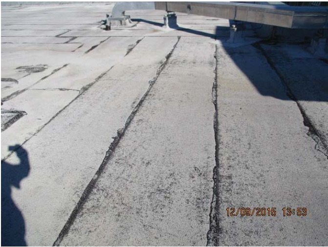
#2 - Predominate Roof Covering - Doesn't Meet 2001 FBC
