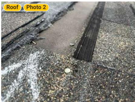
"Close-up of the south-facing slope shows a lifted shingle with the nail partially exposed—classic wind damage consistent with ...
