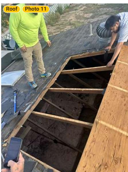
"Roof opening performed by the roofer to expose interior slope conditions—insulation visibly darkened and compromised from mois..."
