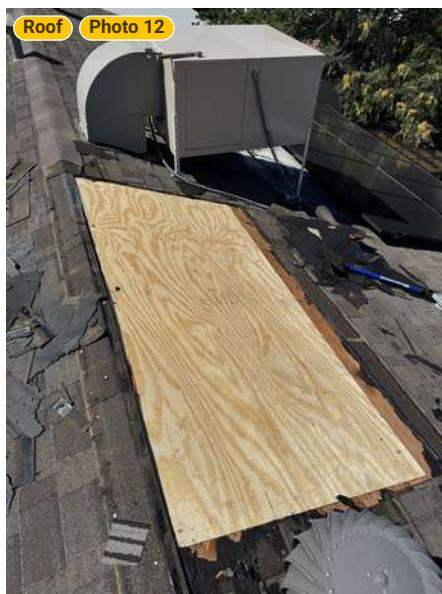
"New 5/8" OSB installed as part of reasonable repairs after the original 3/8" OSB was found to be noncompliant and structurally..."
