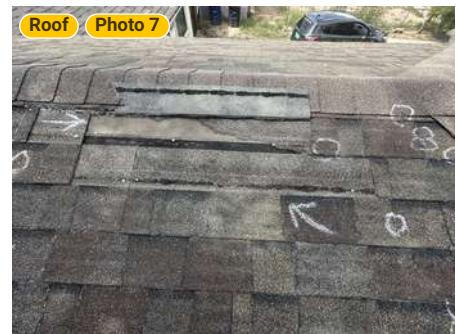
"Carrier-documented wind damage is visible on the south-facing slope, with photo #15 noting 'two wind-damaged shingles' on the ...
