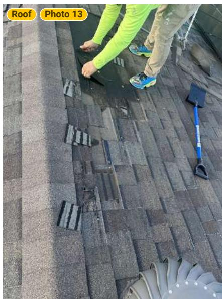
"Roofer performed targeted blading of a rectangular area to locate decking seams—softness between trusses made identification s..."
