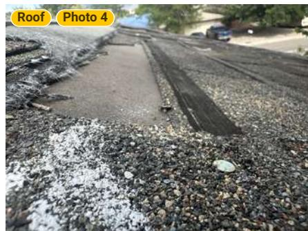
"Shingle on the south-facing slope shows clear uplift with the fastener visibly disengaged—indicative of wind-driven displaceme..."
