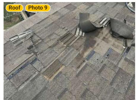
"Roof shown prior to tear-out—wind and hail have visibly compromised the surface with lifted shingles, fractured sealant lines,...
