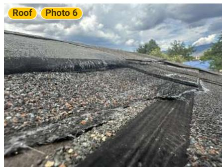
"South-facing slope shows partial shingle displacement—section torn and lifting, leaving the fastener exposed and the water bar..."
