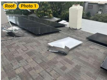
"Wind-blown shingle resting on the skylight confirms active displacement from the roof system—evidence of uplift and seal failu..."
