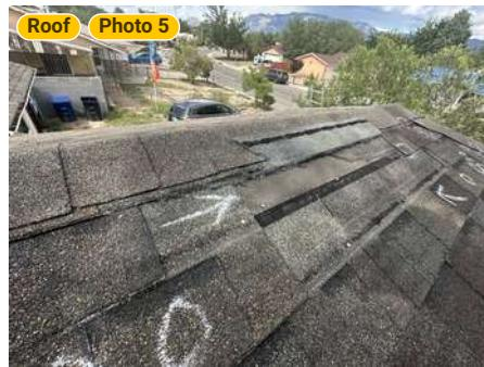
"Carrier photos taken 6/3/2025 by Lee Johnson show wind damage on the south-facing slope, with photo #15 clearly noting 'two ...
