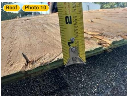
"OSB board shown with tape measure—barely meets the 3/8" threshold, if at all. Material quality is visibly substandard, raising..."
