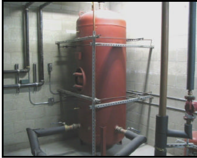
Boiler Storage Tank (Lofts)
