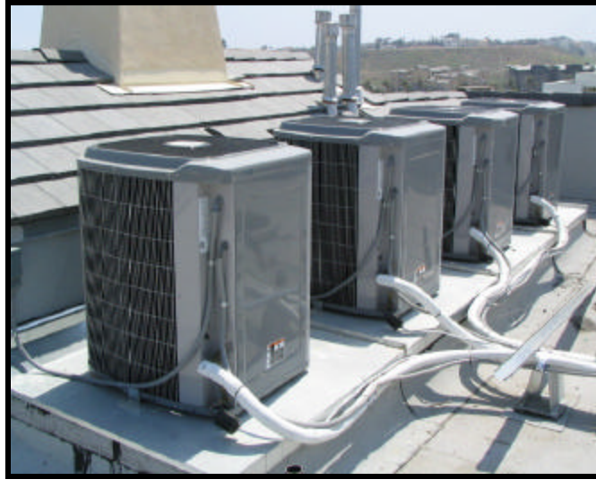
Air Conditioning Condensing Units (Lofts)
