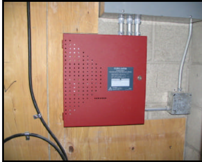
Fire Alarm Control Panel
