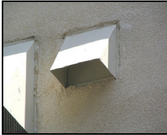
Dryer Vent Terminations
