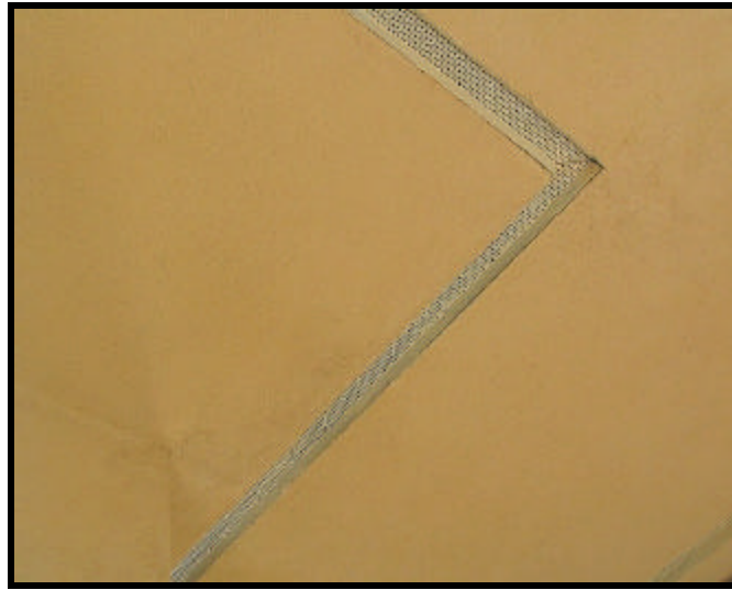
Soffit Vents (Lofts)
