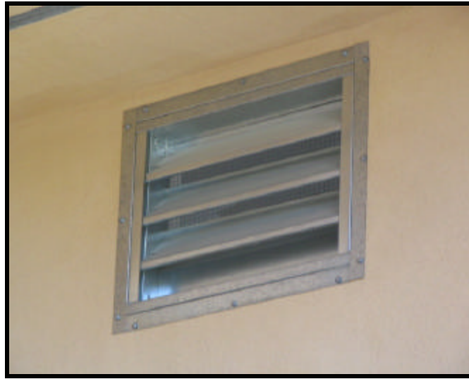
Metal Vents and Flashing
