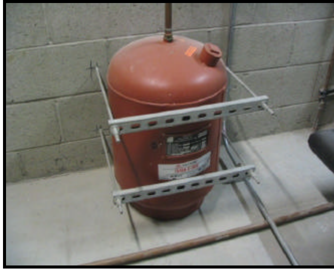
Volume Relief (Expansion) Tanks
