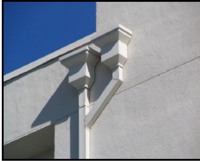
Roof Drains - Scuppers (Park Houses)
