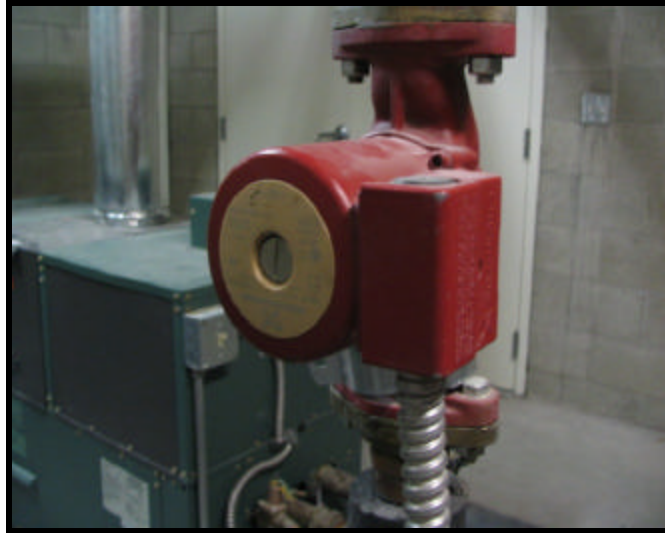
Boiler Recirculating Pumps (Lofts)
