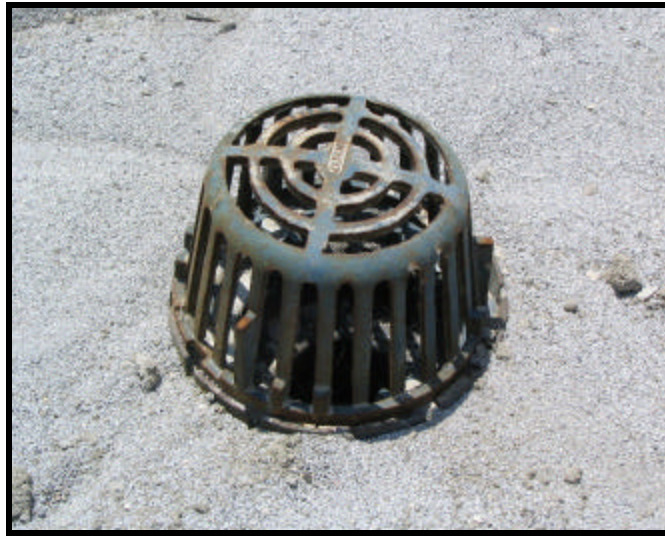
Roof Drains - Standard
