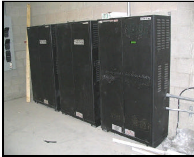
Emergency Battery Backup System
