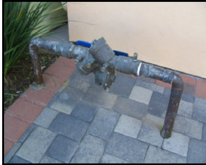
Irrigation Backflow Devices
