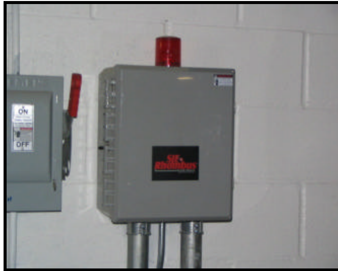
Sump Pump Level Alarms
