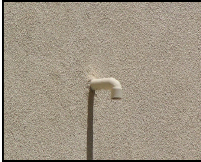
Air Conditioning Condensation Drain Line
