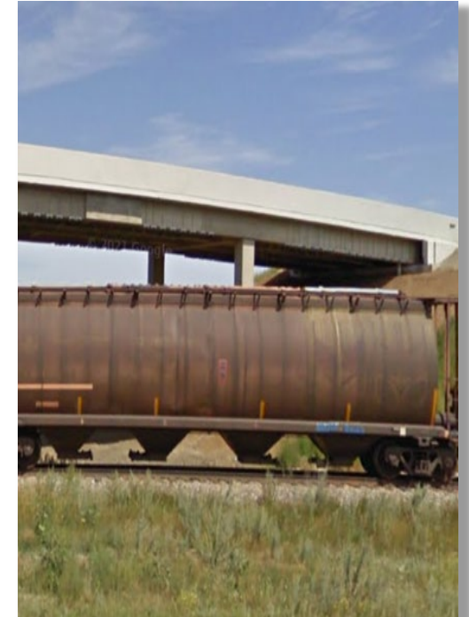
HWY 39 Bridge Overpass Meeting SK Highways specifications
