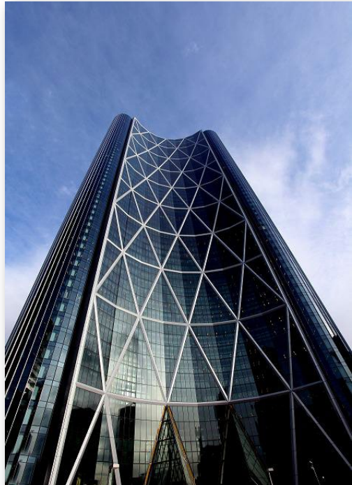
The Bow Calgary Improved pumpability, shrinkage resistance and strength properties allowed for significant project efficiency gains
