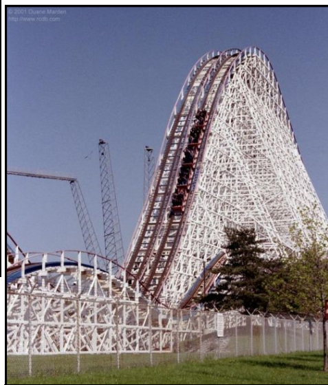
The first hill of the American Eagle is 147 feet tall so riders can coast along 4,650 feet of track without motors or engines. (Frank Prager, Six Flags)
