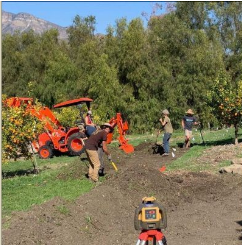
Mama Tree working with Grounded Landworks on a major earthworks installation in spring 2021: a swale, berm, and infiltration basin
