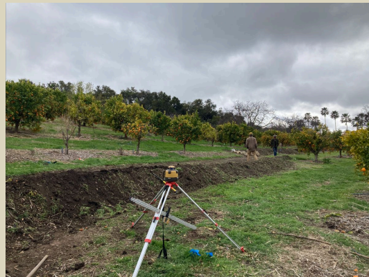
Mama Tree working with Grounded Landworks on a major earthworks installation in spring 2021: a swale, berm, and infiltration basin
