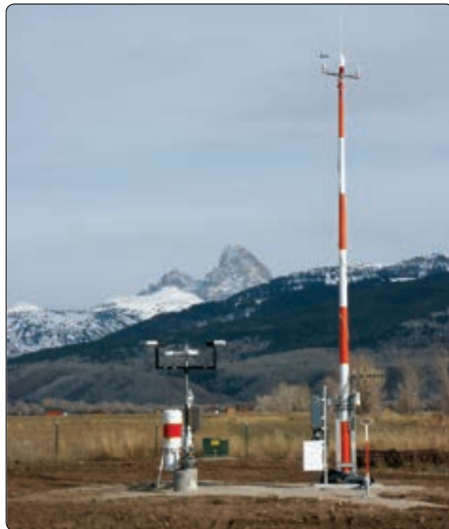
Figure 1-11. AWSS installation at Driggs-Reed, Idaho.
