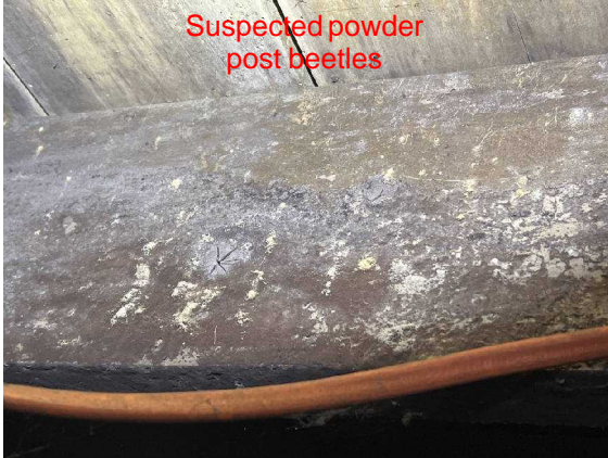
Suspected powder post beetles
