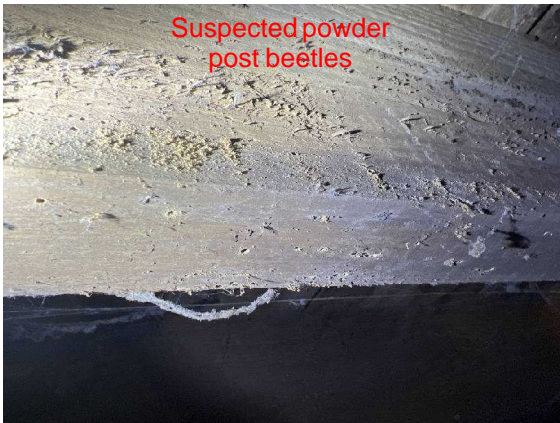
Damaged joist has been repaired but new joist attaches to deteriorating beam
