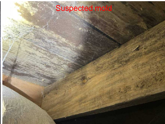
Much of the crawlspace has much newer joists and sub floor
