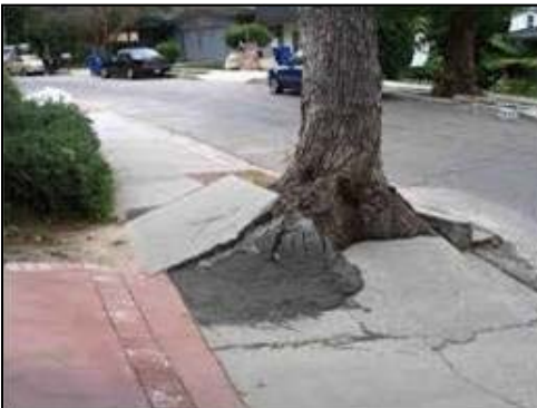
Photo of broken sidewalk from wrong tree planted in the wrong place. Where possible the broken sidewalk can be cut out and the tree planting area expanded by cutting out additional sidewalk as seen in the next photo
