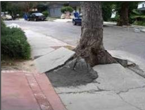
Photo of broken sidewalk from wrong tree planted in the wrong place. Where possible the broken sidewalk can be cut out and the tree planting area expanded by cutting out additional sidewalk as seen in the next photo
