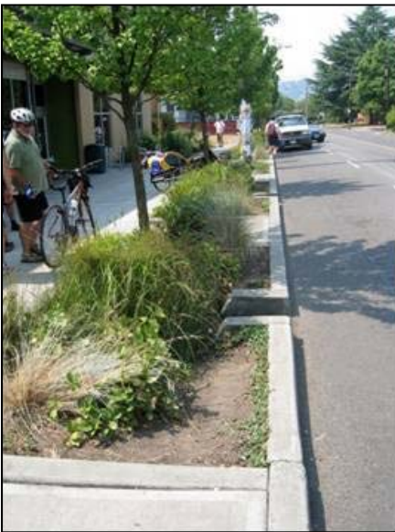
Photo of one example of a Rain Garden where stormwater runoff coming down the street at the curb can be directed into a planting area for use by plants and groundwater recharge
