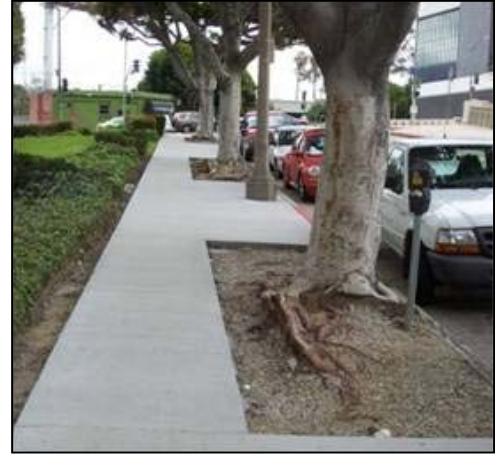
Photo of an expanded tree well that was created by removing broken sidewalk and then cutting out additional sidewalk to expand the tree grow space so roots don't continue to uplift the sidewalk
