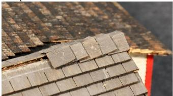
25. Next, fold the 2-tab shingles in half along the center line, so they sit on the peak of the roof.
