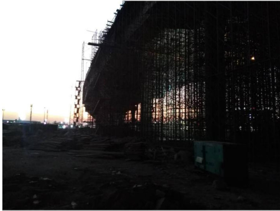
construction site of a new bridge in Alasher microbuses node mobile photo, taken by: Azza Ezzat, 2021
