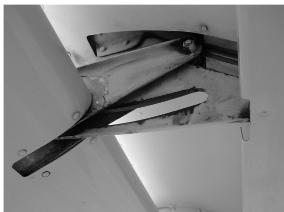
Check for damage to surfaces and flap tracks, freedom of operating linkage and security of all nuts and lockwires.
