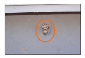
**5.** Slowly open the valve at the water meter. Don't just "jerk" the valve open. Open the valve a quarter turn every 5-10 seconds. This won't "shock" the plumbing lines possibly causing a leak within the system.
