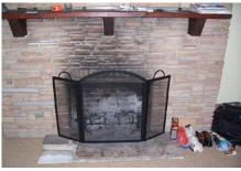
Figure 2. Soot above the fireplace can also indicate dangerous gases accumulating inside the home.
