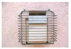
Figure 3. Wire cage installed over direct vent to protect against burns.
