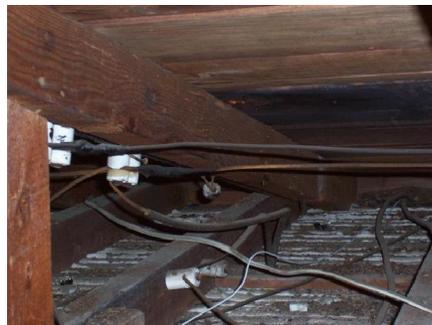
Figure 2. Knob and tube wiring.
