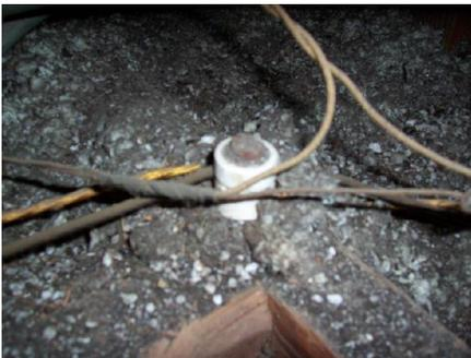
Figure 4. Attic insulation covering knob and tube wires.
