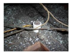
Figure 4. Attic insulation covering knob and tube wires.
