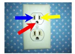
Figure 5. Modern electric outlet showing slots for hot (yellow), neutral (blue), and ground (red) wires.
