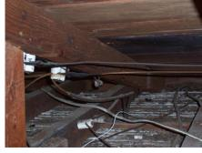
Figure 2. Knob and tube wiring.
