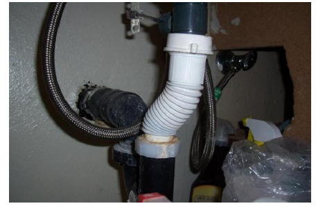
Figure 3. Flexible accordion drain pipe.
